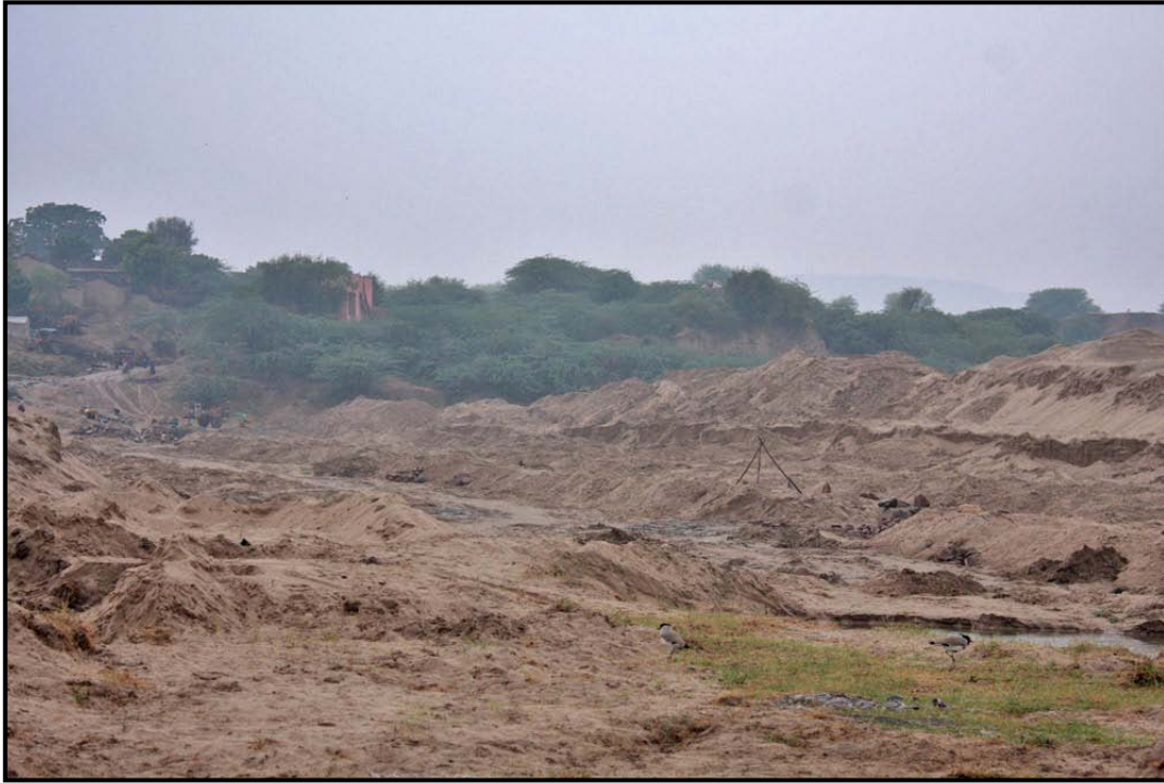
Image: Banas banks under construction for road
