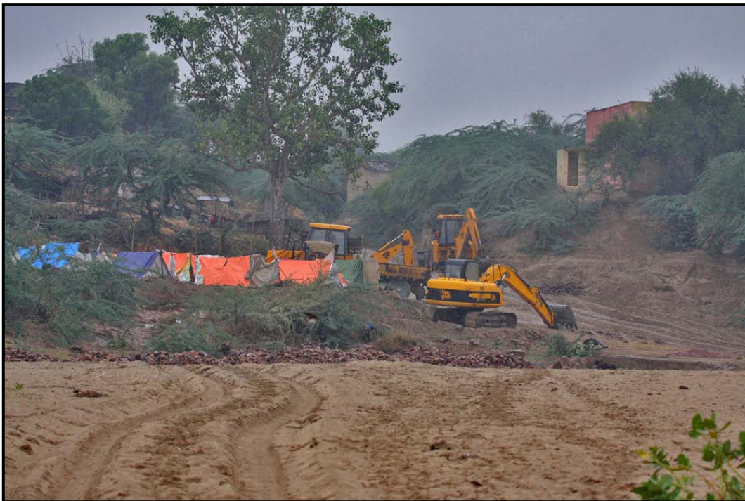
Image: Heavy machinery being used at the site
